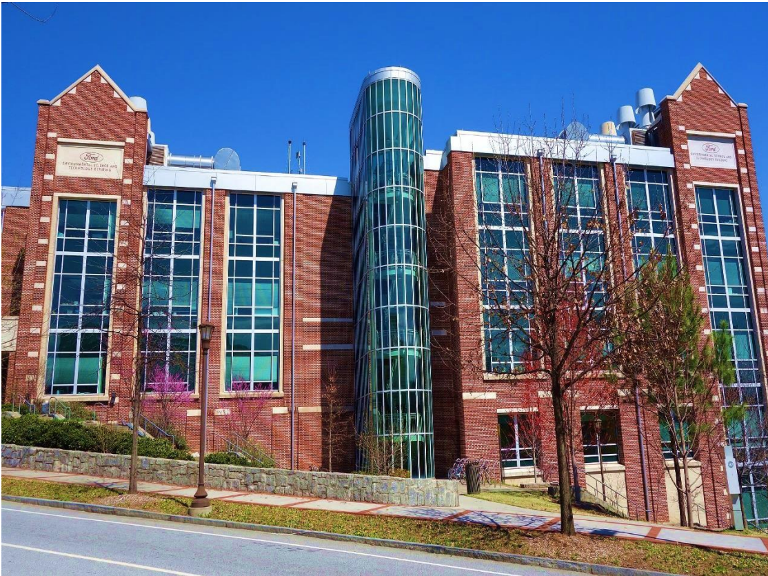
Ford Environmental Science and Technology (ES&T) building which houses the ChBE chair's office
